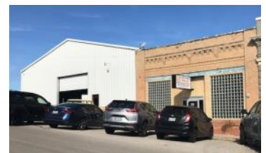
The Mercantile store-front that the Hindmans plan to restore to its original appearance and the more recent warehouse.
