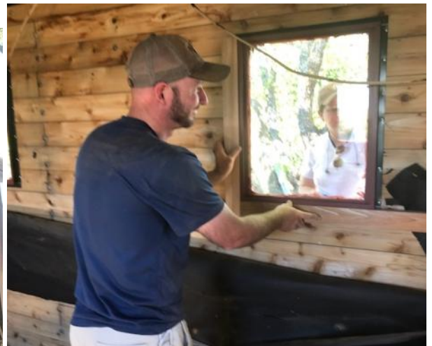
Left, Rosie Haines and Dustin Haines of Haines Craft Construction paint around the new windows. Above, Dustin fits wood trim around the inside of the windows, while Rosie paints outside. Photos by Susan Garry
