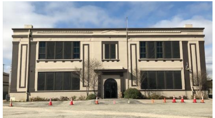
The historic Coupland school building has been painted as part of the construction and renovation project. Photo by Buz Garry
