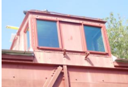
An important part of the function of a caboose--the observation windows around the cupola have been restored.
